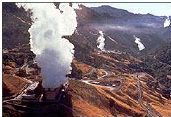
Dry steam power plants at The Geysers in California.
